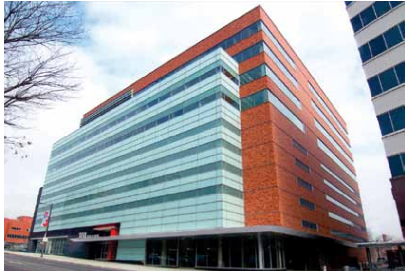
The Wexford Science and Technology Building in Philadelphia, designed by Zimmer, Gunsul, Frasca, uses opaque glass to provide light without glare, making it safer for birds. Photo courtesy of Walker Glass
